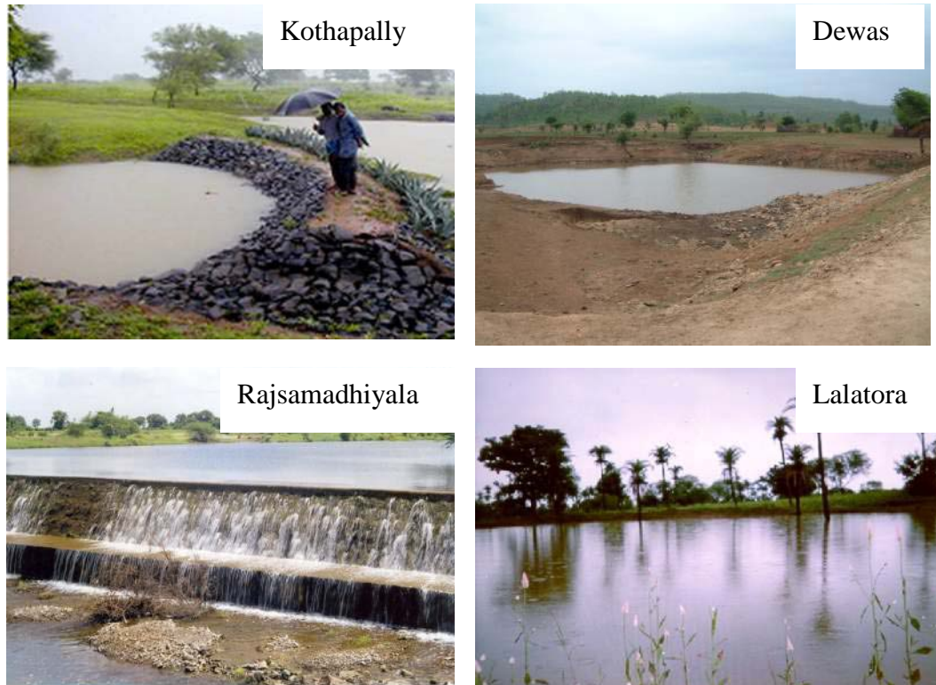
Figure 1. Runoff harvesting structures constructed in community watersheds in India.
